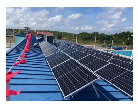
Have you noticed the rooftop panels on the locker room building at the Aquatic Center in Destin? The solar panel array was installed in mid-April, went fully on-line on April 24, and has been turning Florida sunshine into electric power ever since! This 24.09 kilowatt system includes 66 solar panels, all securely attached to the standing seam metal roof, tilted for maximum southeast exposure.
